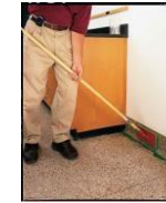
Applying Floor Coating
