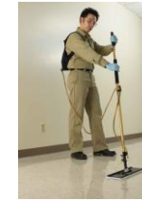
Applying Floor Coating
